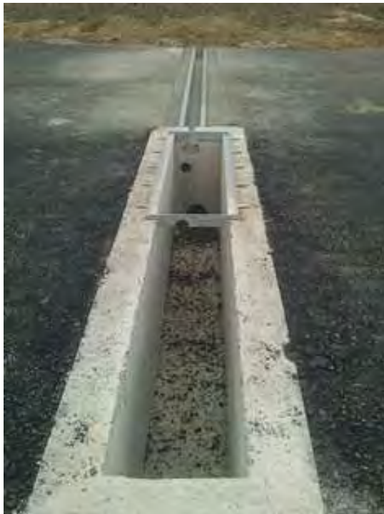
Concrete Case for water obstacle
